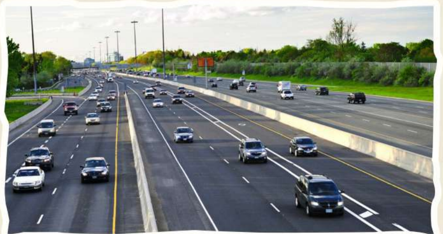
6 Lane GT Road
